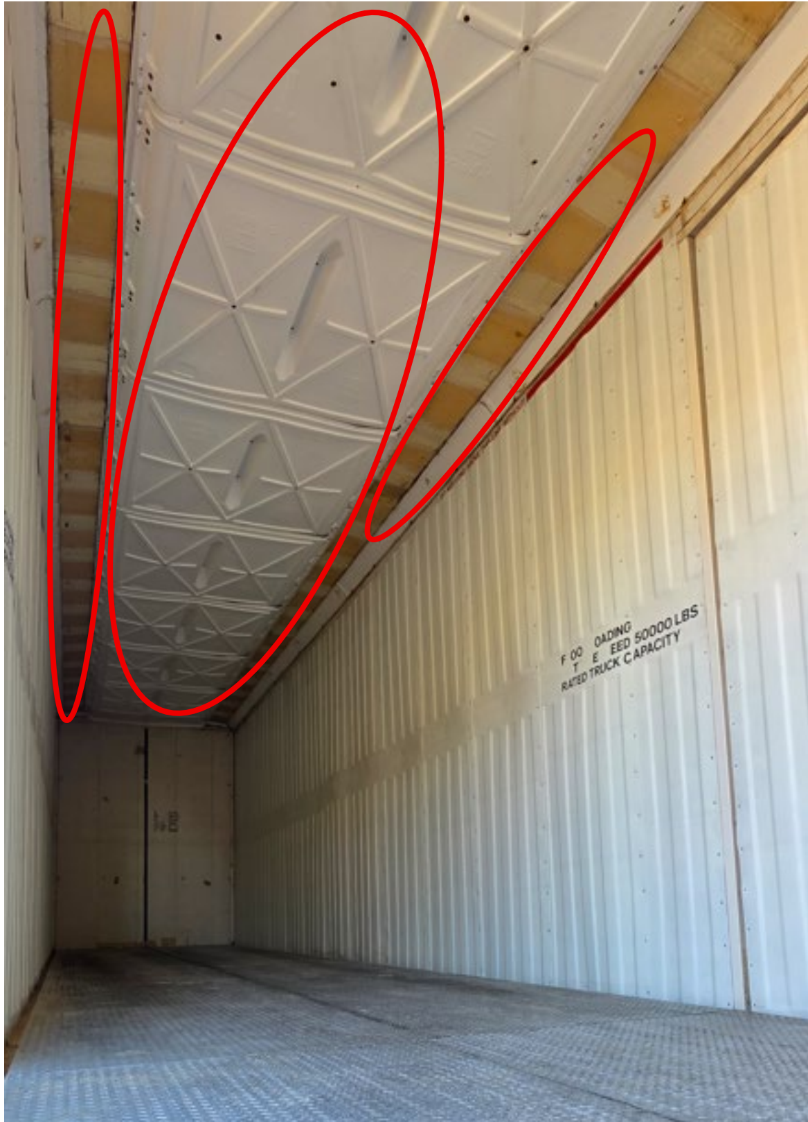
Exhibit D: Plenum (center). Gutters (left and right).
