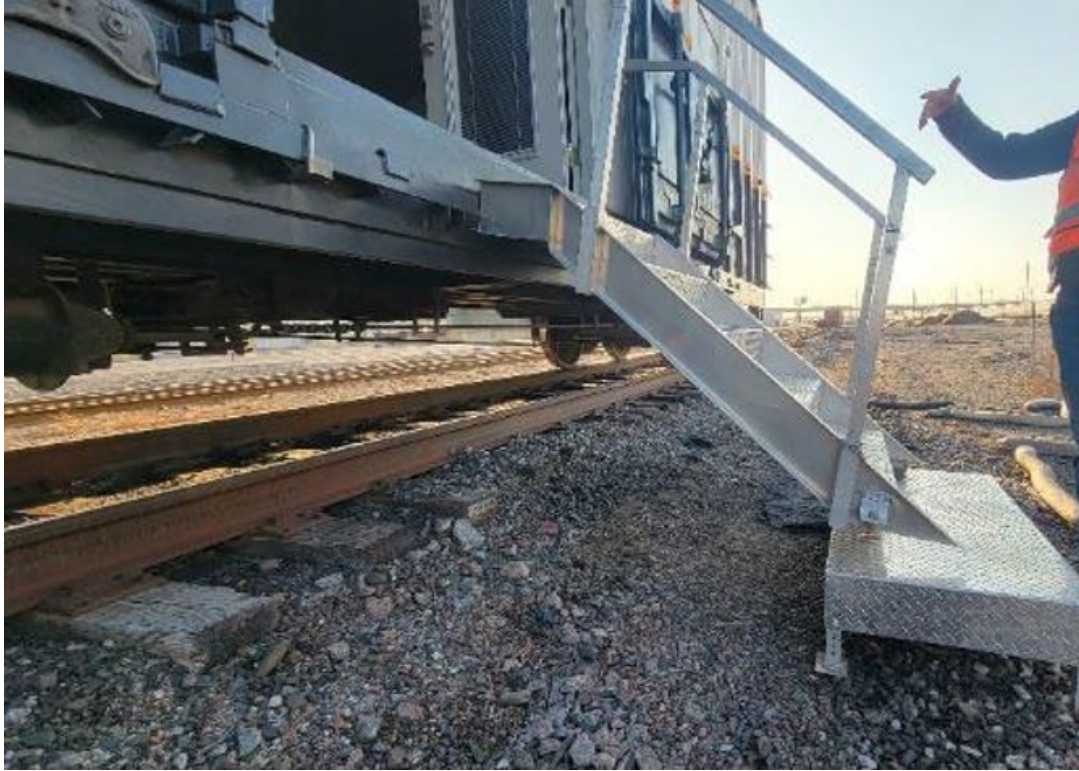
Exhibit F: View of example stair system with handrail.
