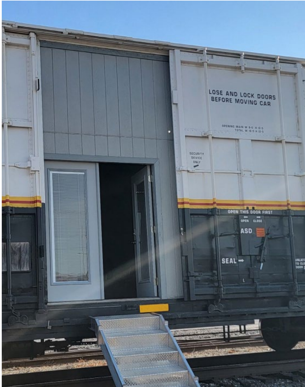
Exhibit E: Finished exterior wall behind plug door opening and at least 96”H by 60”W double-door with built-in blinds.
