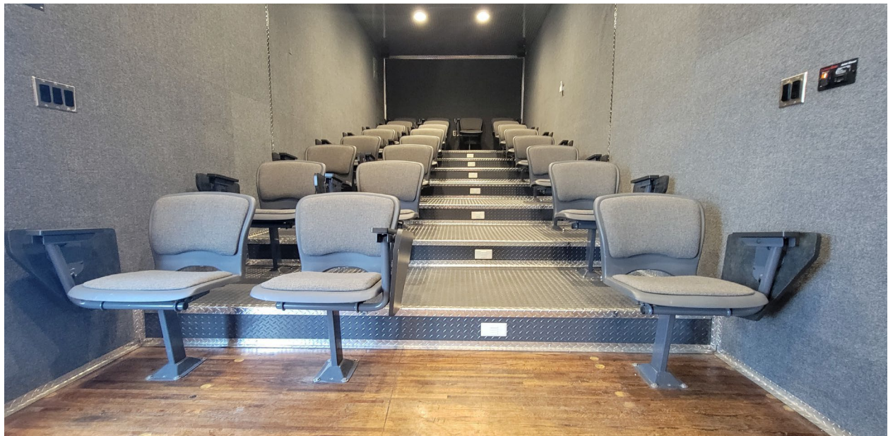
Exhibit D: Shows floor to riser transition, seating/aisle layout, flush mount aisle lighting, rubberized flooring with diamond-plate toe/edge protection trim.
