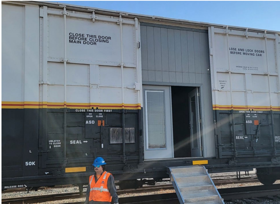
Exhibit A: Example of exterior finished wall behind railcar plug door. 60" double-door with built-in blinds.
