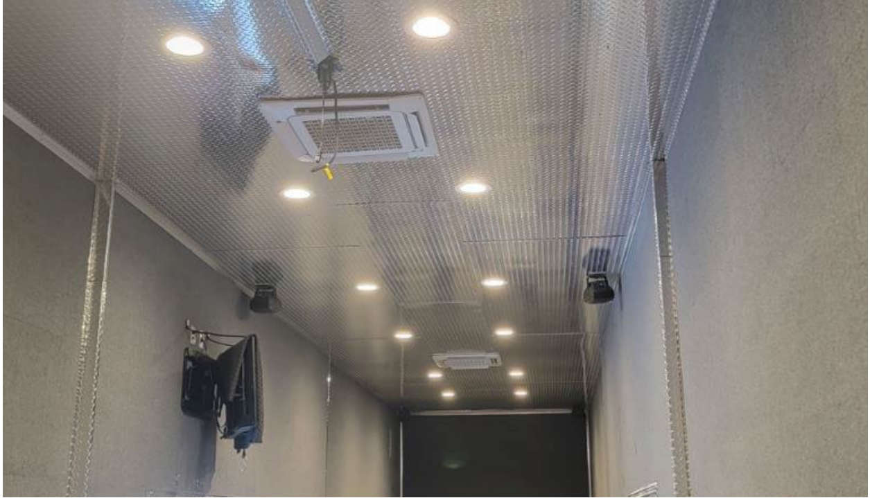
Exhibit E: View of interior finished wall and ceiling materials. Also shown are lights, speakers, HVAC, video monitor, and projector mount examples.
